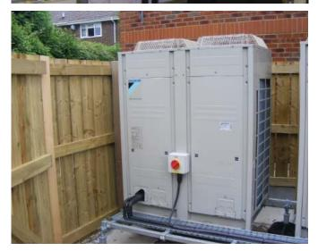
Since the outdoor and indoor units are connected using small diameter refrigerant piping (as opposed to larger water pipes used in other systems), only a small service shaft is needed to accommodate the system's flow and return refrigerant connections from the outdoor unit. This means the system can be retrofitted into buildings with existing service ducts or old shared boiler flue shafts.
